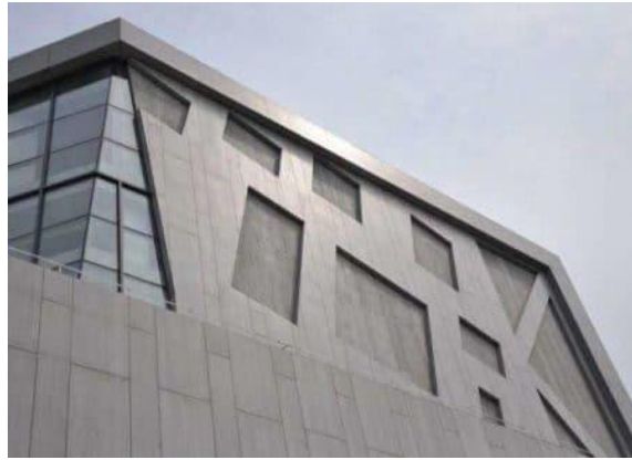
Fig 22: Exterior Siding with Fiber Cement Boards
