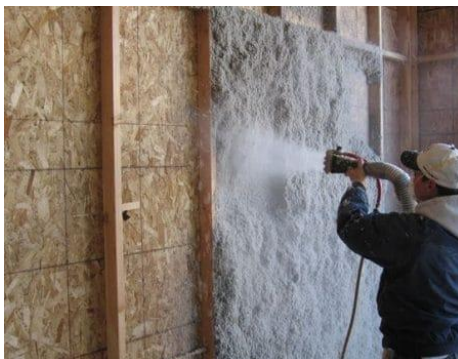
Fig 16: Installing Cellulose Insulation
