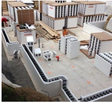
Fig 5: Insulated Concrete Forms
