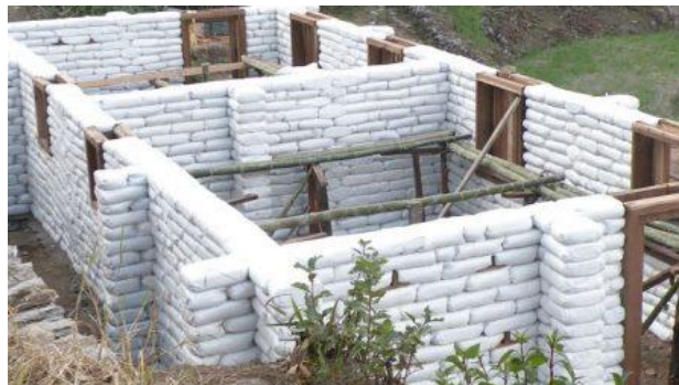
Fig 8: Earth Bag Walls
