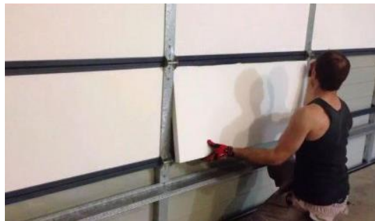
Fig 18: Installation of Polystyrene Foam Sheets
