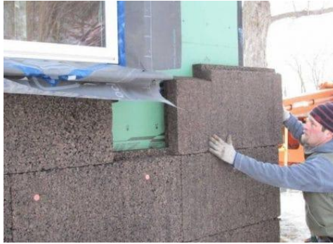
Fig 17: Installing Cork Boards
